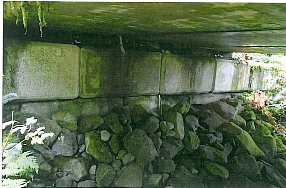
CK-2353 Left Abutment
