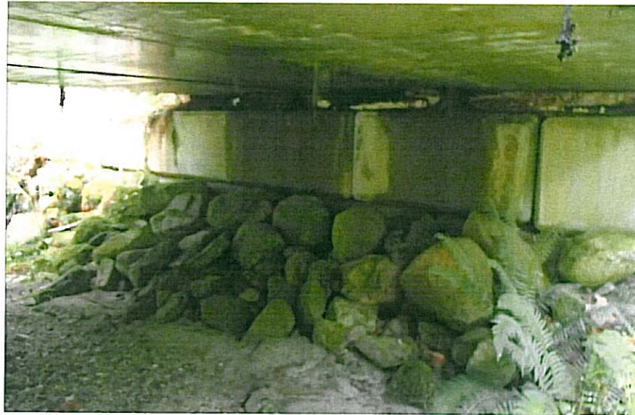
CK-2353 Right Abutment
